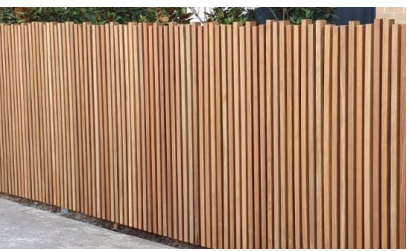
1.5m Timber Batten Privacy Fence
