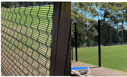
2.1m Perimeter Mesh security fence
