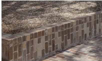
Recycled brick retaining wall
