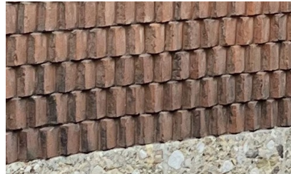
Brick and terrazzo seating bench utilising recycled pool tiles and mosaic from site
